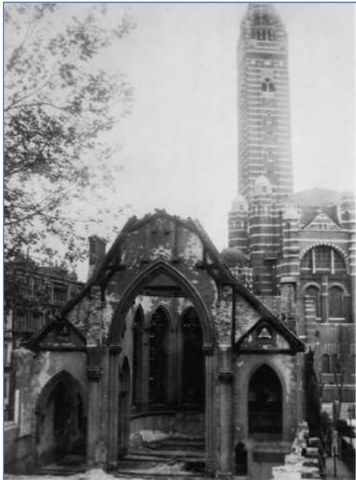
The gutted remains of St Andrew's Church, Ashley Place, after a direct hit in late 1940, showing the proximity of the bomb to the Cathedral.
